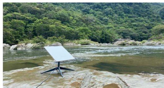
Installation of Starlink
