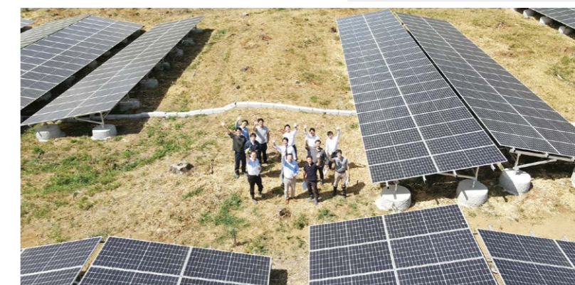
Exterior view of the power plant in Kumagaya City, Saitama Prefecture
